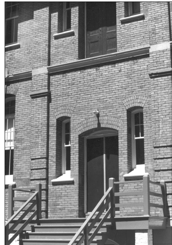
THE MICHIGAN STREET ENTRANCE BEFORE RENOVATIONS
